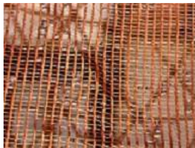
Fig. 3. Interior Plastic Mesh
